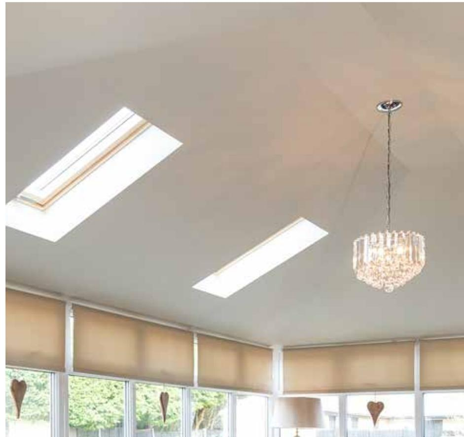
The internal surfaces of your Equinox roof are finished with insulated plasterboard creating the look and feel of a conventional home extension.
