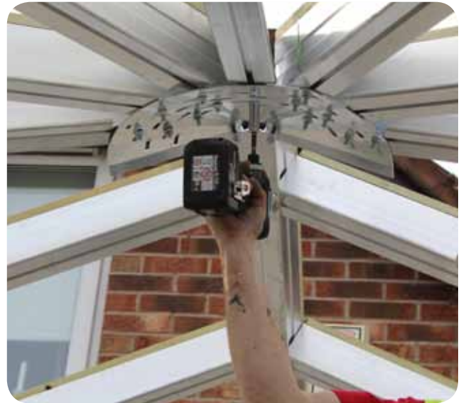
1.14 Secure hips and standard rafters into ridge-end plate using 13mm bolts supplied.
