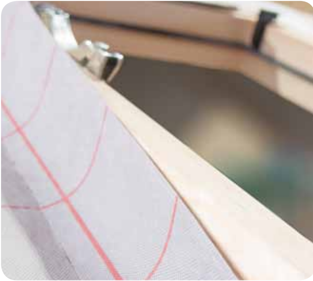
3.5 Drop the roof window into place. Ensuring the breathable membrane covers the outside of the frame.
