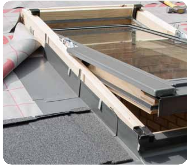
3.6 Install the roof window following the manufacturer's instructions.
