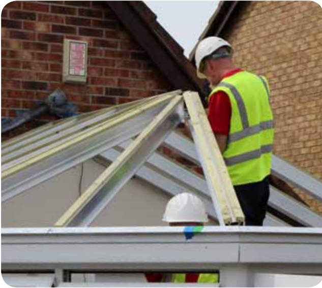
1.13 Slide hip rafters onto the ridge-end plate, affixing with 2 x M8 13mm x 25mm bolts (supplied) to complete the hip section.
