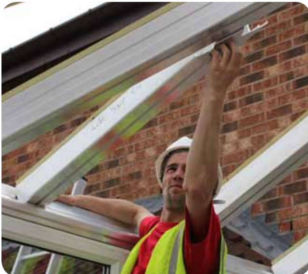
1.15 Secure the jack rafters to the hip rafters with the brackets that were attached in Step 1.12 with M8 13mm x 25mm bolts (supplied)
