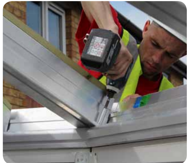
1.16 Secure hips and jack rafters onto the ring beam using M6 10mm x 30mm bolts supplied.
