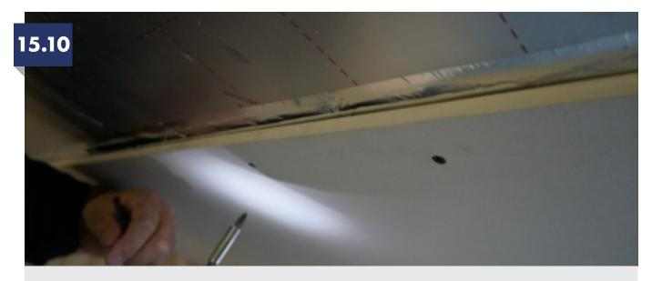
Once all joints are sealed install the 12.5mm plasterboard sheets over the PIR insulation. Use the 100mm drywall screws to fix the plasterboard ensuring they pick up on the battens behind the insulation. Ensure the drywall screws are installed at least 10mm from bound edges or 13mm from cut edges and the screw heads are flush with the board face. Drywall screws should be installed at 300mm centres.
