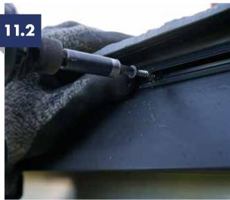
Using the supplied grey painted stainless steel screws fasten the seal to the eaves, repeat along the entire length at 300mm centres.
