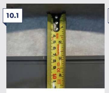
The roof window cut out through the ply is required to be 70mm above the required SlateSkin panel as shown below.
