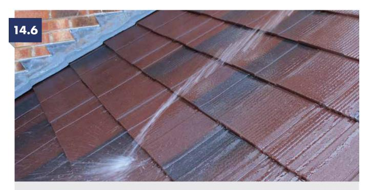
We advise carrying out a water test for all tile types using a hose to represent heavy rain fall. The water should fall vertically, do not direct the water up under the tile joints. This should be done before any internal work commences.
