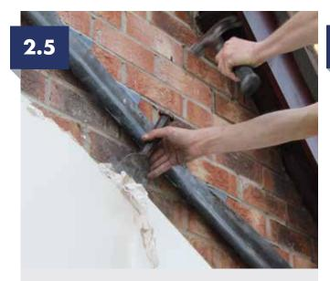
If necessary, tidy up any plaster so the new gable rafters go up to the host wall.
