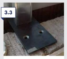
Position the assembly in its correct location. The support post should be flush to the underside of the ring beam to offer full support to the roof.
