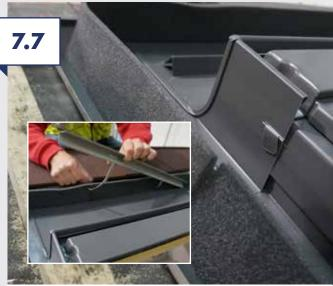
Fit the top flashing kit, remove and discard the tile support angle.
