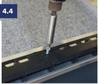
4 Install all fascia vents along all sides of the ring beam using 4.2x38LG self-drill screws through the pre-set holes identified in the moulding. At corners, ensure vents are cut tight to each other.
