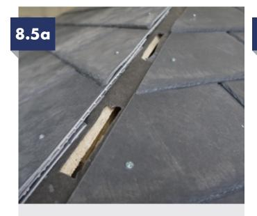
Where two facets meet over the hip, the tiles need to be cut and mitred leaving a 30mm maximum gap. Cut rectangular slots up the hips 200mm x 20mm sections though the HR membrane to allow breather space.
