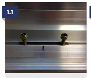
All the M6 double and single studs should already be set in position on the ring beam. Check the position of the studs and that they are all there. Slide in additional studs if required.
