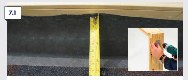
Position the roof window 85mm above the immediate tile below the roof window position, marking out roof window perimeter cut ply/insulation. On the roof window fixing brackets, flatten the small location tang (inset picture) so the brackets sit flat directly onto the ply. Fix the roof window ensuring the felt is lapped up the sides of the roof window.
