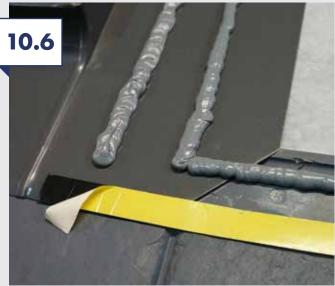
Run two generous beads of Soudal Fix All High Tack adhesive sealant (or equivalent) down the side flashing trays as shown.
