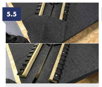
Fix the metrotile hip vent moulding to the 19x38 hip battens using 4.2x16LG screws, then use a hip end cap to position and centralised, using the inner edge of the batten as a guide, mark a reference line on the tile to enable positioning of the battens later.
