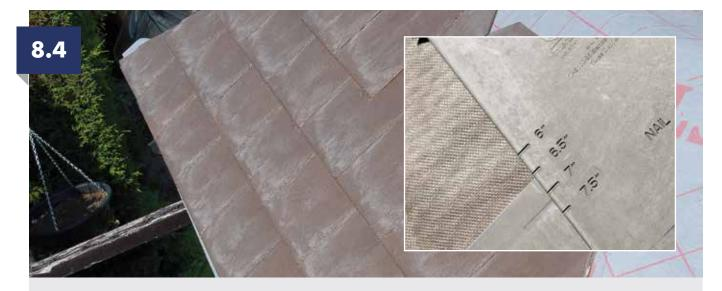
For the next row of tiles, check the lowest pitch on the roof, then set the tile overlap using the gauge shown on the side of the tiles. This overlap should be used for the whole roof.
