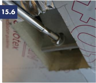
If tie wires have been installed, cut two insulation sheets so the joint is in line with the tie wire, then mark out the tie wire bracket location and cut away the minimum amount of insulation.
