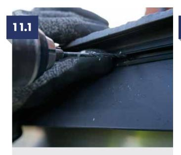
Holding the CRS8480BK seal in position to cause compression under the tile, drill a pilot hole using a 3mm drill through the seal, eaves tray and OSB roof sheets
