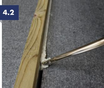
Use an appropriate fire retardant expanding foam to seal any 3mm or larger gaps present between the styrene and the aluminium structure
