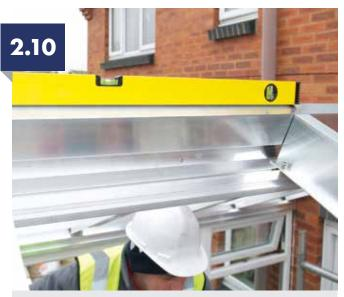
Check the height and level of the ridge. Ensuring rafters are aligned. Tighten all nuts in the ridge and ring beam. Tighten jack rafters and hips at this point. Ensure ridge height is the same as paperwork supplied.
