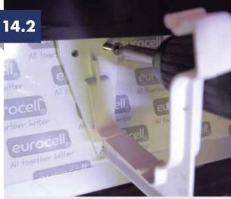
Fix the gutter brackets into the ring beam using self-tapping screws at maximum 600mm centres ensuring protective tape is peeled back first.
