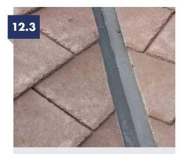
Mitre the composite slates so they finish 25mm from the valley centreline as shown above. Slateskin tile sheets will be supplied pre-cut to the required size.
