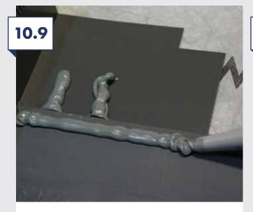
Run a bead of Soudal Fix All High Tack adhesive sealant (or equivalent) across the top of the panel ready for the next side flashing tray to be installed.
