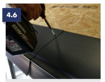
Once the 18mm OSB3 is fully installed, fit the eaves guard around the edge of the roof with a minimum of 50mm overlap and mitred to each other at any corners.
