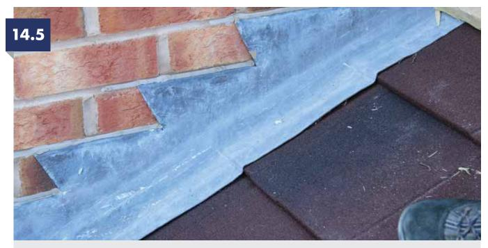
If existing lead is in good condition and appropriate length for the new roof construction, reposition it to complete the external installation. If lead work requires replacing use code 4 lead and ensure the vertical drop and tile coverage meeting appropriate industry guide lines.
