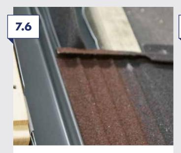
Continue fitting the tiles around the roof window. Note the foam does not need cutting down now the vent is fastened directly to ply. When fastening tiles down fold excess foam away from the roof window. Ensure cuts up to the flashing kit ridge are square and neat.
