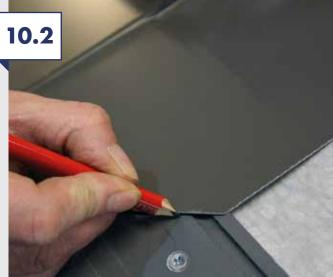
Position the bottom flashing kit and mark the width onto the panel.
