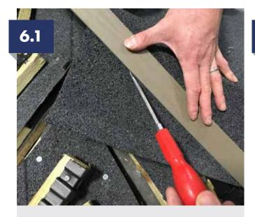
Following section 5 until the last ridge tile, starting at one of the outer hips, cut the last ridge tile so its projects past the crown point. Using a straight edge scribe a line down the ridge centre line and a line from the crown point to the lower tile intersection point.
