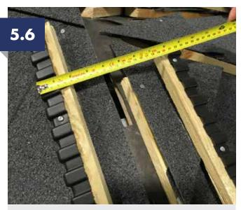
At the crown point use a ridge profile to set the width or set the width of the vent moulding to 240mm, ensuring the centreline aims to the crown point. If the roof has been supplied with a standard crown capping use this to correctly position the battens. Mark the tiles to the inside of the battens for reference later.
