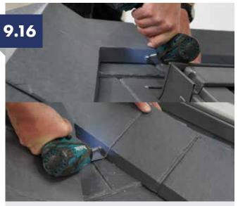
Position and fix the ridge crown caps using the painted grey stainless screws supplied.
