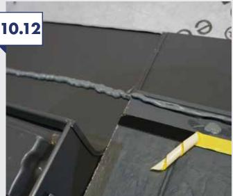
Continue the bead of Soudal Fix All High Tack adhesive sealant (or equivalent) across the flashing hood as shown. It may also be necessary to flatten the upstand slightly on the top of the flashing hood.
