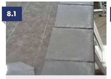
For the first tile course, the tile height requires to be cut to 305mm from base. If the roof section being tiled is up to a single host wall, start tiling from the wall. If the roof section has hips, gable ends or host walls at both sides then start tiling from the centre of the roof section. The starter tiles should be fixed in the marked locations using the supplied 4.2x38LG self-drill screws and positioned so the tiles have a 30mm overhang from the eaves guard.
