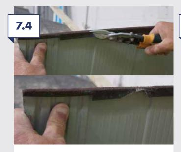
Offer the next tile up and mark where the transition from tile to flashing kit is, cut this away using some aviation snips as shown below.
