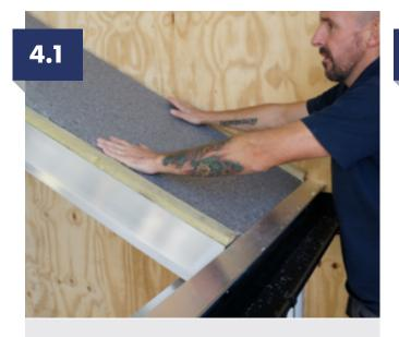
Once all of the framework for the roof is assembled and tightened, install the pre-cut 100mm styrene insulation. Ensure the styrene is fully seated down to meet the base of the rafters.
