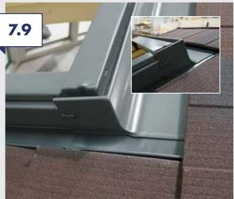
Fit the upper tile(s) and nail or screw the tile in a couple of places into the batten above the flashing kit to secure the front edge. Finish the screws/nails off with Metrotile touch up kit. Note Photo shows a 780mm roof window, if 980mm is fitted then tile will required cutting around roof window.
