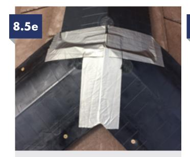
Once mitred/scribed together use butyband to seal the joints on as shown below.
