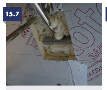
Fill the void with an appropriate expanding foam to fully cover the bracket. Leave the foam to set and trim away any excess before fully covering with PIR foil tape.
