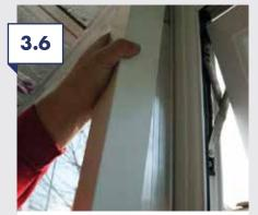
Now the support post is fixed in it's correct position, measure and cut the capping trim to size. Fit the capping trims and repeat the process until all support posts are fitted then re-fit or replace the window cills.
