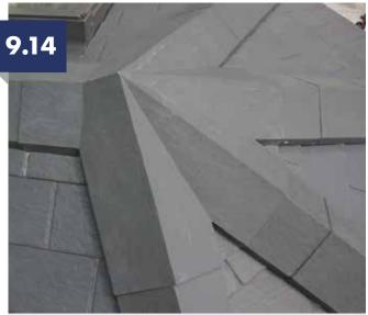
Check the fitment of the crown cap, if all ridge positions are acceptable remove the ridge cappings and fix the battens down fully at 300-400mm centres using 4.8x32mm self drilling screws.
