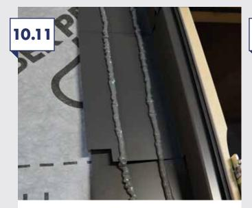
Install the side flashing trays and the top flashing hood to the manufacturer's instructions and install the next SlateSkin panel as previously described.
