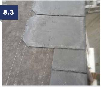
The next row uses full tiles and should be cross bonded with the below starter row. The tiles have fixing location information on them.
