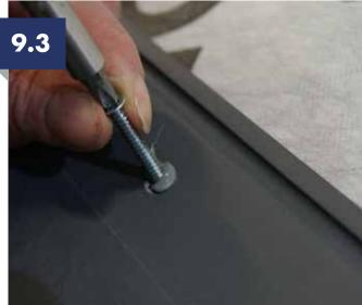
Fix the panel to the roof ply using 4.8x32mm self-drilling screws supplied though the pre-drilled holes. Apply Soudal High Tack adhesive sealant (or equivalent) into the hole before fixing. Ensure the torque is set low and then adjusted to ensure the panel is not deformed.
