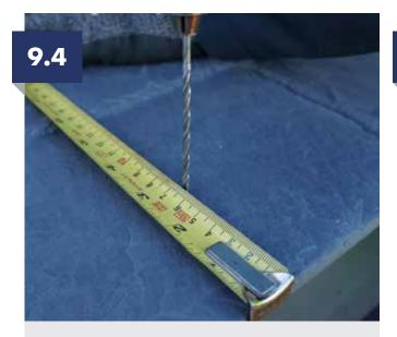
Using a 3mm drill a pilot hole through the panel, plywood and aluminium support 65mm back from the face of the SlateSkin panel. Perform this every other tile impression on base of the starter tile only. (Do not repeat this on any other panels further up the roof slope)
