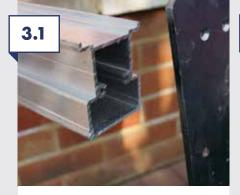
Cut the support post to size, measure the distance from the underside of the ring beam to the internal brickwork below and deduct 5mm for the support plate.
