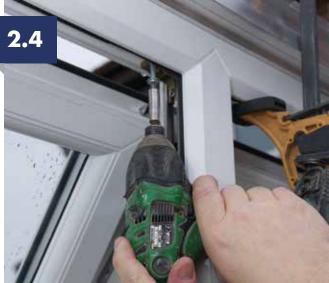
Once the ring beam is in place, screw up from the frame using 5.5mm self-drill bay pole coupling screws (not supplied) to secure 300mm centres, ensuring you keep 150mm away from any welded frame joint.
