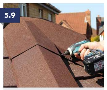
Complete the tiling by fitting the ridge moulding. Use repair kit to cover screw heads.
