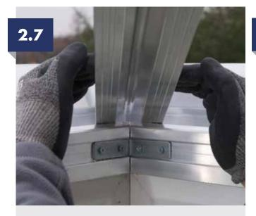
Once the ridge is in place, locate the hips. Aligning the centre of the hip with the corner of the frames. Ensure the centre line of the hip strikes through the centre line of the ring beam bolt slots.
