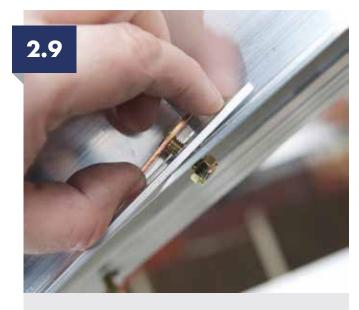
Locate any jack rafters on the ring beam and studs. Use single studs supplied to fix the top of the jack rafter to the hip. **Do not** fully tighten the nuts.
