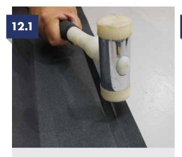
Using a nylon mallet, flatten the valley tray sides against a hard surface.
