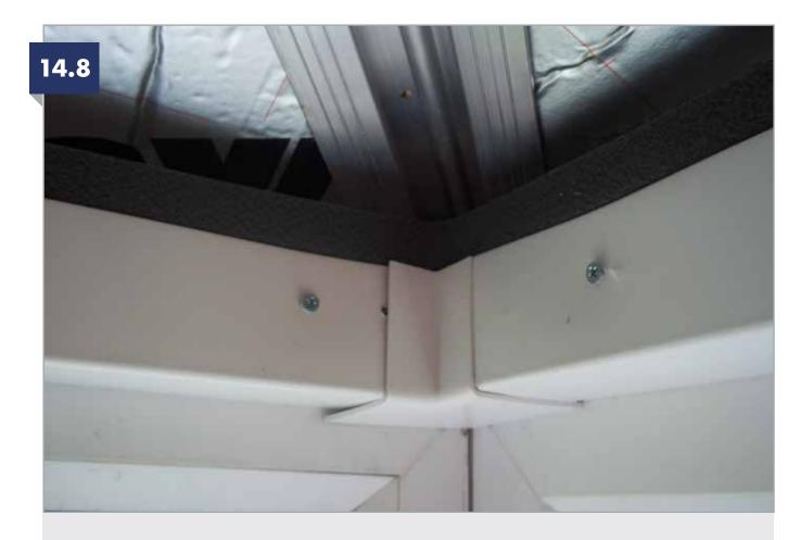
Once the RA6060 internal trim has been installed, fit the appropriate corner trims using an appropriate glue/adhesive.
