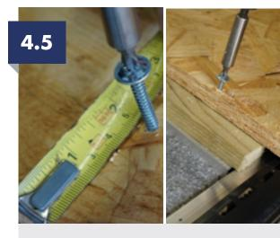
Cover the entire roof with the pre-cut 18mm OSB3 boards, refer to the supplied plan to identify the correct locations. Fix the bottom boards to the ring beam using 60mm self-drilling screws (supplied) 50mm from the front edge, every 300mm. Fasten the remaining edges and along any intermediate rafters using the same fixings at 300mm centres. Top boards should be fastened along the ridge or wall plate.
