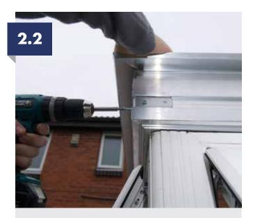
Continue locating the ring beam using the internal and external Brackets and the self-drill screws (supplied).
