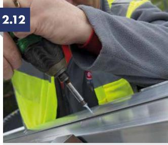
Ensure jack rafters and hips are correctly aligned. Set hips in position using the self-tapping screws supplied.
