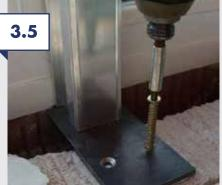
Drill and fix the support plate to the internal brick/block work with suitable fixings.
