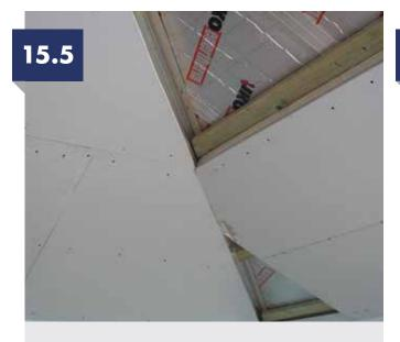
Proceed from the bottom of the roof working upwards, cutting the shapes from the stock sheets to fit the roof faces.
