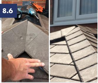
Install ridge tiles using 60mm fixings with appropriate overlap and marked fixing locations. At the ridge intersection the tiles will require mitring together to suit the roof geometry. Any joints can be sealed using appropriate colour sealant.
