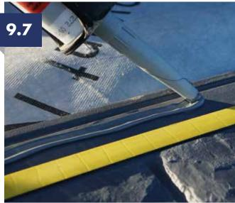
Ensure the tile is dry and clean, then apply an 8-10mm bead of Soudal High Tack Fix All adhesive sealant just below the recess channel of the panel ensuring the adhesive sealant covers any fixing screws.
