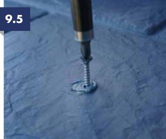
Using a countersink bit, countersink the panel until 10mm in diameter. Apply soudal fix all high tack adhesive sealant (or equivalent) into the hole, then fix using grey painted stainless steel screws being careful not to over torque and deflect the panel. Wipe any excess sealant away.
