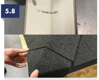
Install the hip end caps and then the ridge tiles by fixing through the vertical upstands into the side of the batterns, note the ridge tiles are slightly wider on the base to allow overlap onto the previous tile, usually the base of the tile has a printed reference number at the base of the tile but check the width at both ends. Ridge tile should have 110mm overlap.
