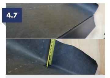
Cover the roof with HR membrane (supplied). Ensure the starting edge is to the front of the felt tray, do not extend the membrane past this point. Minimum horizontal overlap of 225mm for below 15 degree roof pitch and 150mm for 15 degrees and above. Lap membrane up host wall a minimum of 75mm. If additional roof membrane is required ensure it is HR type membrane (Non-breathable membrane) and is suitable for the pitch and location to be installed.
