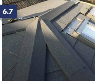
Use the glue and dust kits (supplied) if additional cover of the joins is required.
