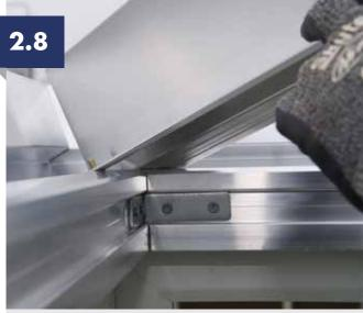
The hips are a two-part component and locate into the ring beam and rest on the wok (to be bolted later).
