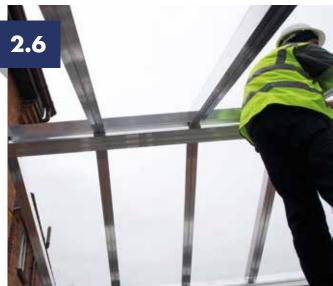
Using the pre-positioned studs, locate the rafters in the ring beam and ridge in the marked positions. **Do not** fully tighten the nuts. Again, check the alignment of the frames.
