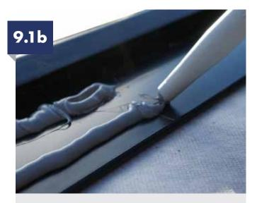
If an end bar is present, prepare the verge tray by running two generous beads of Soudal Fix All High Tack adhesive sealant (or equivalent) until just past the height of the SlateSkin panel.
