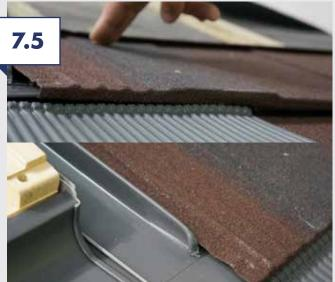
Where the tile rides over the flashing kit slightly bend down the tile hook and press down the lead flashing, this allows the tile to hook under the steel flashing and shingle to the side, ensuring the front edge is fully restrained.
