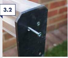
Attach the support plate to the support post with the screws provided.
