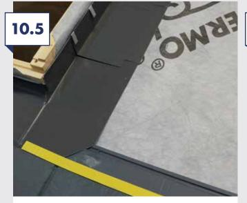
Install the side flashing trays and position 50mm above the top of the next SlateSkin panel. Run the HTAF tape over the bottom flashing as shown.
