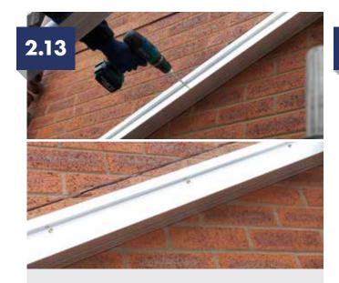
Fix gable rafters (at 400mm centres) to the back wall using suitable fixings (not supplied).
