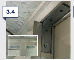
Using the supplied angle brackets, fasten the ring beam to the support post. 2 angle brackets are required on each support post.
