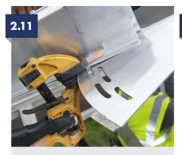
Clamp the 'wok' to the hip. Use the M6x50LG bolts, nuts and washers supplied into the pre-drilled hole and bolt together. Do not fully tighten.
