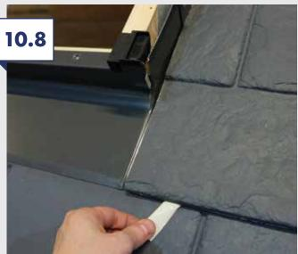
Position and fix the panel as previously described, the bottom of the panel should be in line with the flashing tray.
