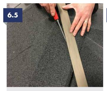
Position and fix the ridge tile battens so that the height of the ridge tile is sufficient to ride over the hip tiles at the crown point.
