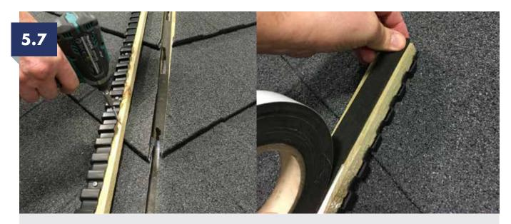
Apply the metrotile expanding foam to the underneath of the battens and then align with the reference marks and fix using 4.2x38LG self drill screws at each tile base. Noting the tape may take a few hours to expand and fill voids.
