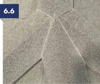
Lay the ridge tile 20mm past the crown point and scribe a line to the outer tile intersection point, then trim the ridge tile. At the tip cut back to the crown point and fold down to restrain the tips of the hip tiles. Fix the ridge tiles to the battens through the outer edges.
