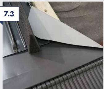
Fold the flashing kit over as shown below, this directs any water blown sideways down. The lead skirt can also be cut the same width as steel base for neatness (Optional). Ensure a vertical batten is positioned at the side of the flashing Kit, not underneath.
