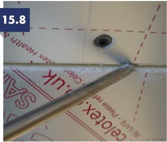
Ensure any gaps in between the insulation are filled with an appropriate expanding foam.
