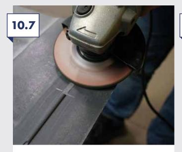
Cut the SlateSkin panel and position 2-5mm away from the side flashing. Then grind the location nib away on the underneath of the panel to allow panel to ride over bottom flashing tray. Use appropriate dust mask when cutting and grinding the panels.
