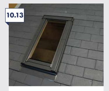
Install the SlateSkin panel above the roof window, 980mm high roof window shown. The SlateSkin panel above a 780mm will require notching around the flashing hood.
