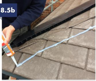
Before applying the hip/ridge masters run a generous bead of silicone down both sides hips and ridge, ensuring the silicone is set back from the outer edges of the hip/ridge masters.
