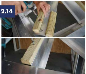
Install continuous 19x38mm battens on to the top face of all rafters using 4.2x38LG self-drilling screws. All hips, ridges, wall plates and valleys to have 300mm sections of battens fitted 100mm apart to allow airflow. (Some battens may be pre-installed by the supplier)
