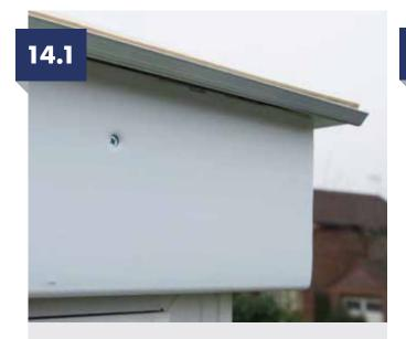
Install capping board by positioning the first gutter bracket and marking its location. The screw will then be covered by the gutter bracket. These steps can be done before or after the drip tray and membrane are installed.
