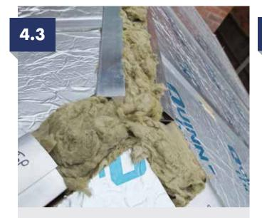
At the crown and ridge of the roof, insert cavity insulation (Supplied) between the aluminium. Also insulate the void at the bottom of the hips where it meets the eaves beam.
