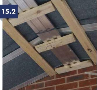
Fix horizontal battens onto the base of the ridge at 600mm centres, or alternatively fix to rafter battens lower down to create a vaulted ceiling.
