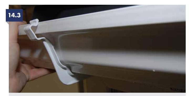
Fix the guttering into position on the gutter brackets, taking care to seal the external angles. Affix corner trims onto fascia boards. Install gutter corners, stop ends and outlet.
