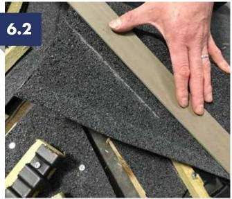
Using tin snips, cut the ridge tile upstand at the lower intersection point and fold the tile up to allow the tile to seat down, then mark another line 20mm parallel to the original one.
