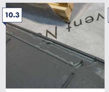
Run two generous beads of Soudal Fix All High Tack adhesive sealant (or equivalent) in between the flashing tray marks as shown below.
