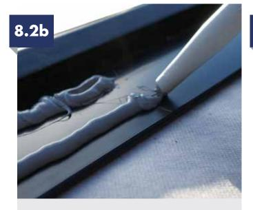
If an end bar is present, Install and prepare the verge tray by running two generous beads of Soudal Fix All High Tack adhesive sealant (or equivalent) underneath each tile.
