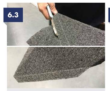
Cut the tile to the outside line and then fold the tile up along the first line to create a valley gutter. Tip; when using tin snips cutting in the correct direction will not leave a white line down the tile surface.
