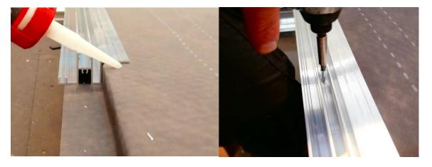
11. Insert Qlon gasket into Aluminium seal rails and trim to length, then Install the horizontal seal rails as shown below using 4.2x38LG screws. Ensure the aluminium seal rails are flush with the internal aperture. Insert Qlon gasket into Vega glazing bars and trim to length.
