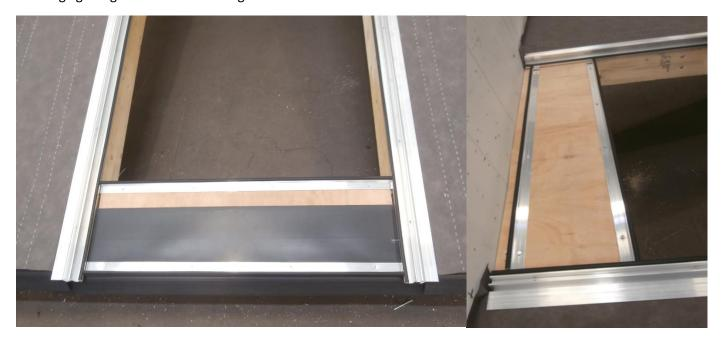
12. Roof tiling can now commence up to the Vega glazing bar, run a generous bead of sealant down the Vega glazing bar before laying each tile. Ensure the tiles are cut to leave a 5-7mm gap.
